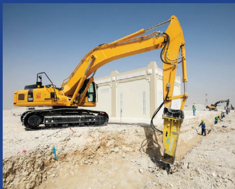
Galfar Al Misnad is home to a large and specialized Plant department. 1672 units of fleet and equipment enable the safe, reliable, and cost efficient implementation of Galfar's vast business operations in Qatar.
